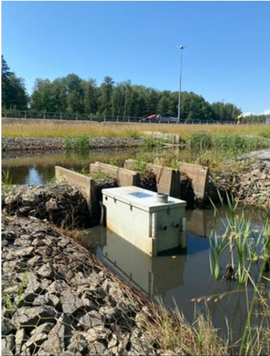
*Figure 58 The main retention pond and outlet with final filter.*
