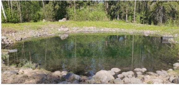
Basin 1: influent from drainage system (2019). Water quality was monitored as taking a composite sample. Settling tank in drainage system is located near influent pipe.
