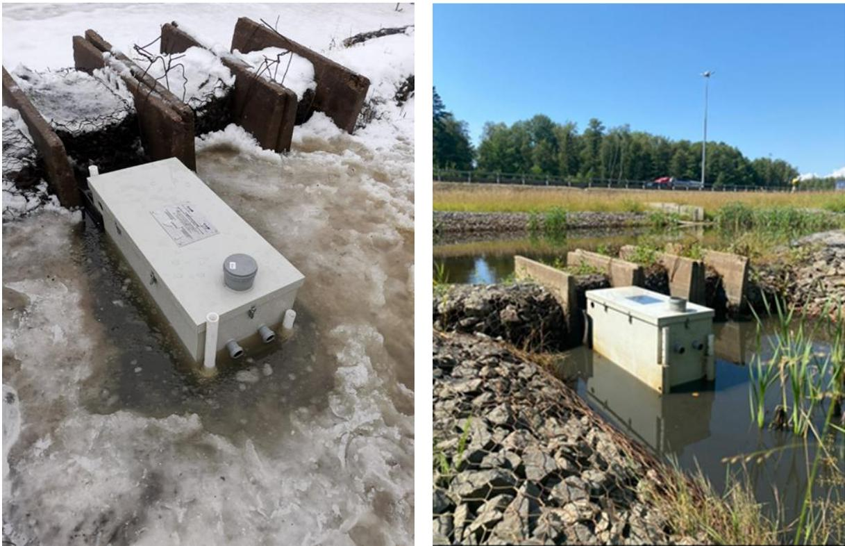
Figure 100 Installation of filter in the stormwater retention pond.
