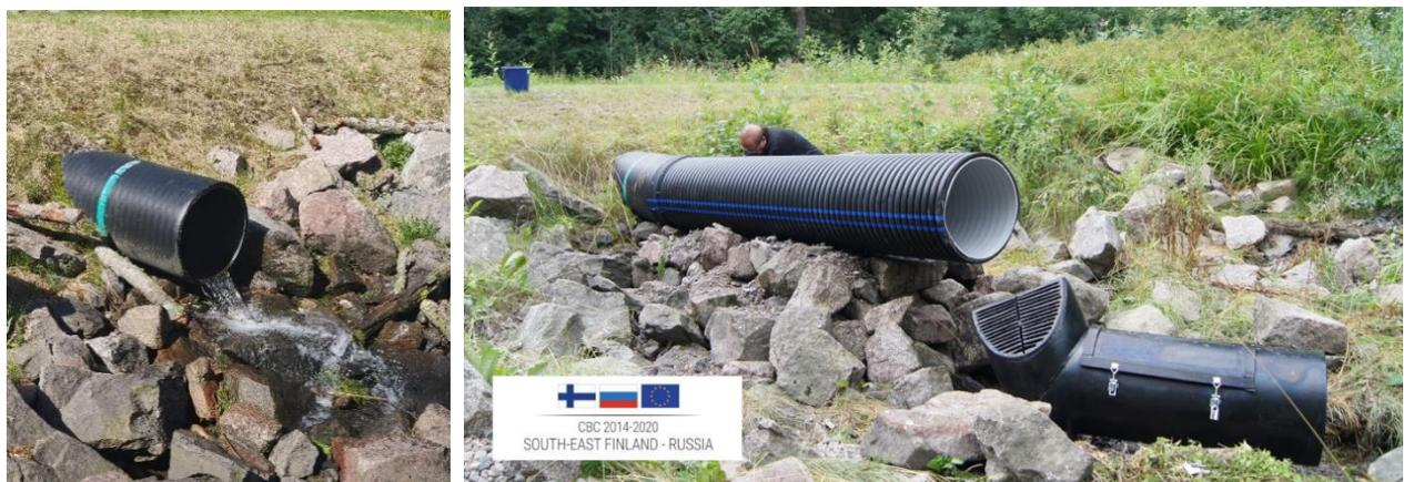
Figure 44 Outlet pipe from 1<sup>st</sup> basin before and after the filter installation.
