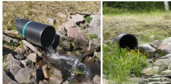
Outlet from Basin 1: filter location, water quality and flow monitored as single weekly samples
